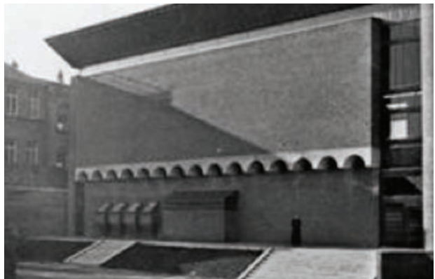
Right: Cast concrete arches at St Patrick's Kilsyth
