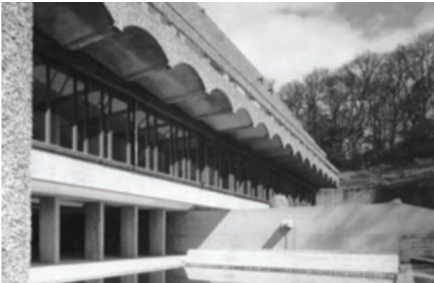
Left: Cast concrete arches at St Peter's Seminary Cardross
